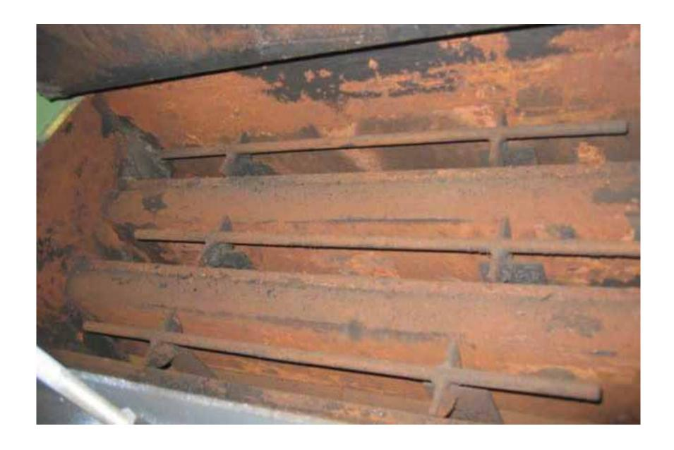
Heat exchanger flue way, heavily coated with corrosive material left over from burning miscanthus
