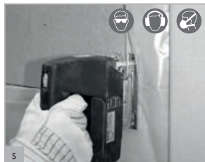
5 Make the opening. NOTE: Bearing elements must not be weakened! IMPORTANT: follow the safe working notes on page 35.
