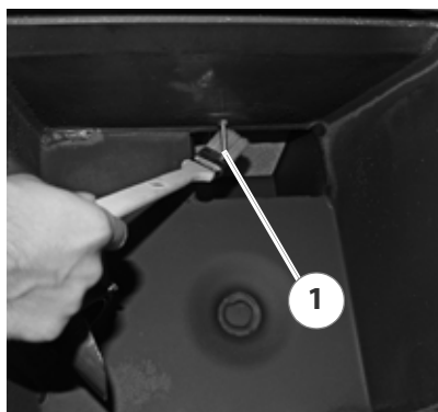
Figure 7/5 - Cleaning the combustion chamber temperature sensor
