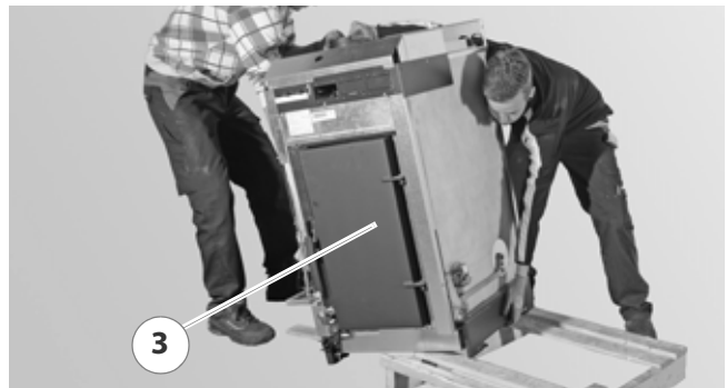
Figure 4/7 - Removing the transport pallet - 2
