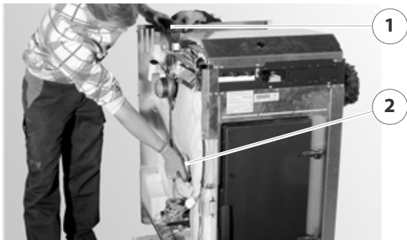
Figure 4/7 - Removing the transport pallet - 2
