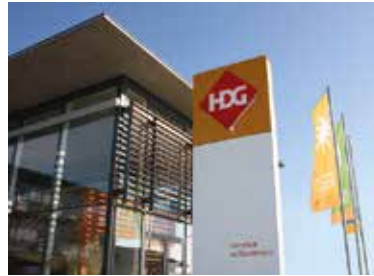
Completion of the administration building
